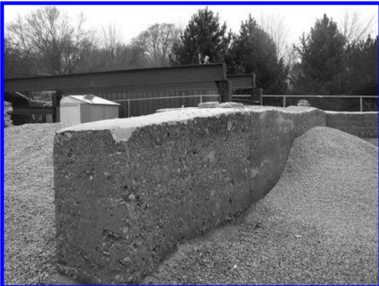
FIGURE 27. Rammed earth wall.
