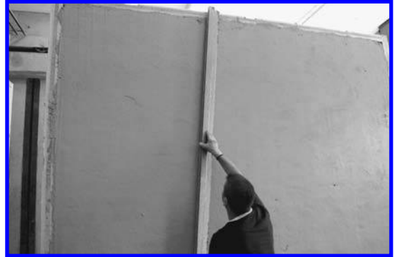
FIGURE 6. Finishing the surface of a ModCell panel (courtesy of Prof. Peter Walker).
