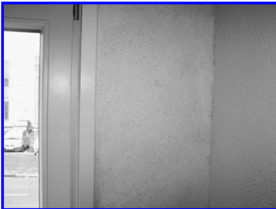
FIGURE 18. Exposed hemcrete surface on interior of building.
