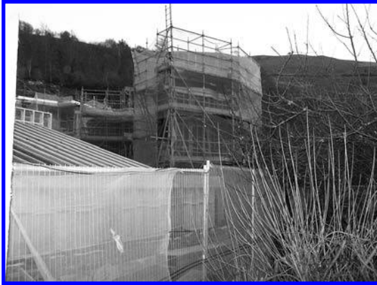
FIGURE 29. Formwork for rammed earth walls of WISE lecture hall.
