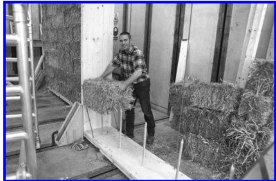
FIGURE 3. Stacking bales within Mod-Cell panel (courtesy of Prof. Peter Walker).
