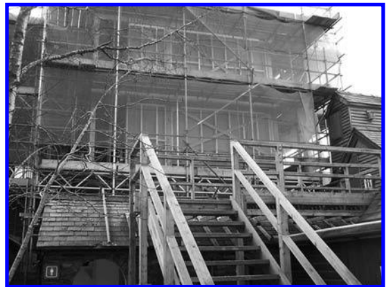
FIGURE 24. Residence walls under construction.
