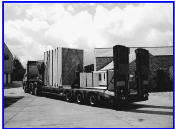
FIGURE 7. Transporting ModCell panels (courtesy of Prof. Peter Walker).
