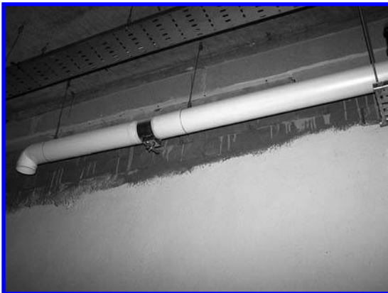
FIGURE 30. Unfired clay bricks being used for partition walls in Lime Technology office.
