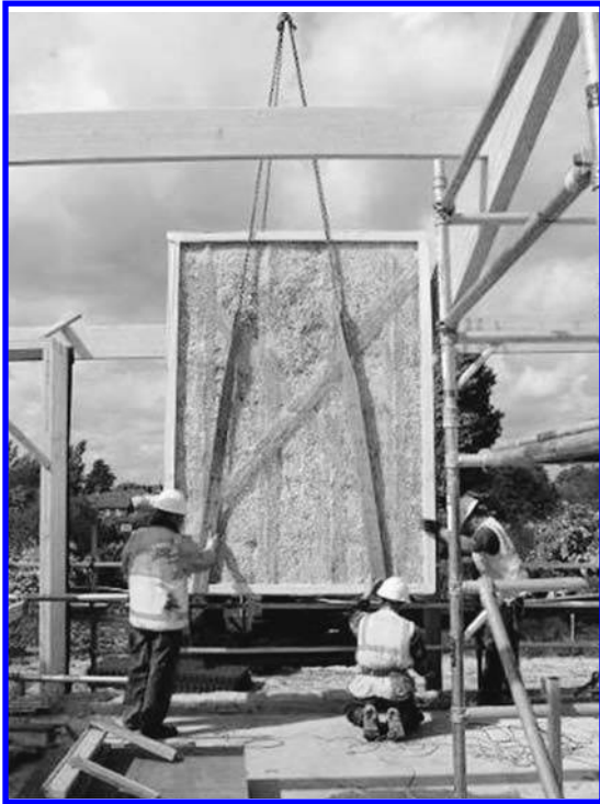
FIGURE 8. Craning ModCell panels into place.
