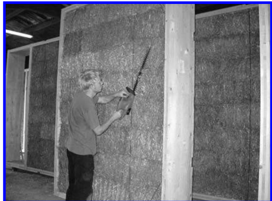
FIGURE 4. Trimming of straw (courtesy of Prof. Peter Walker).
